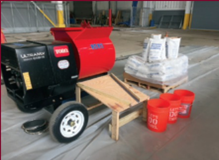
Mortar Mixer, Aggregate and Buckets
