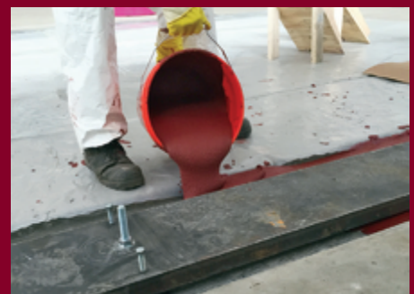
Chockfast Red HF being Poured
