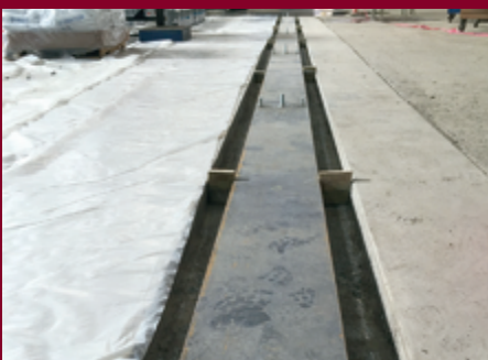
Forming Blocks in Place
