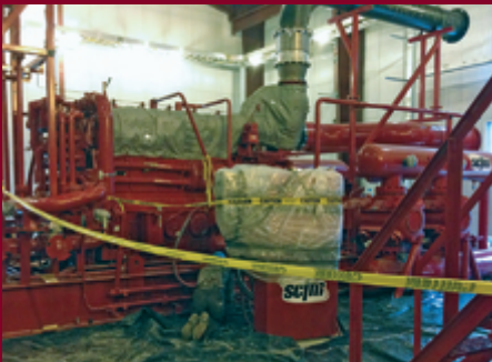
Skid Package being Prepped for Epoxy Grouting
