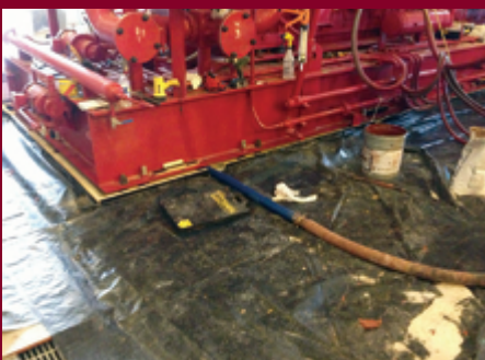
Chockfast Red HF being Pumped
