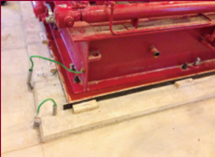
Wood Forming for Compressor Skid Package
