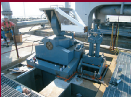
Positioner with Chockfast Orange Installed
