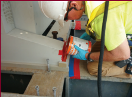
Pouring Chockfast Orange Under Positioner
